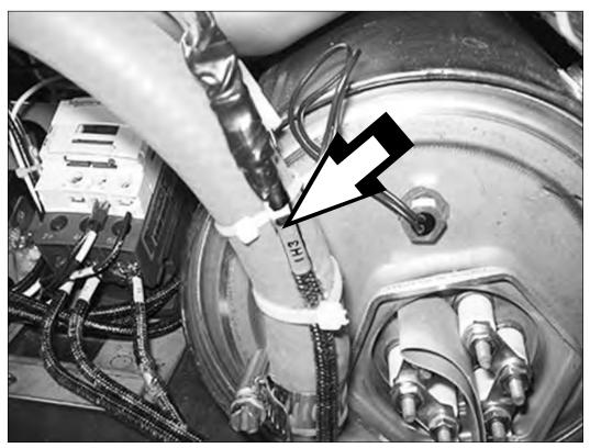
The three phase booster wire (1H3) is cable-tied to the hose adjacent to the booster tank.
